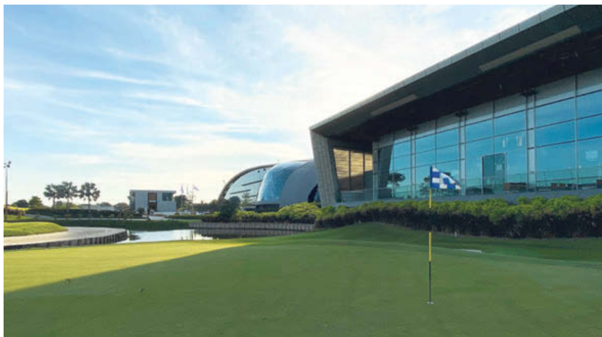
(Left) Exterior of the clubhouse.
