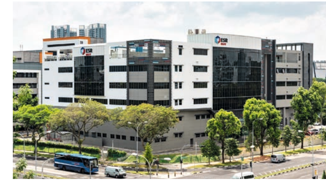
FROM ABOVE LEFT: T30 Marsiling Industrial Estate Road 8; 30 Toh Guan Road (General & Light Industrial).
